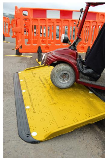
In accordance with a site specific risk assessment (SSRA), appropriate safety clothing should be worn when placing, securing or moving boards and ramps. This may include safety footwear, gloves & high visibility clothing. Works should be designed to ensure that no person is required to work underneath a footway board, driveway board or road plate.
