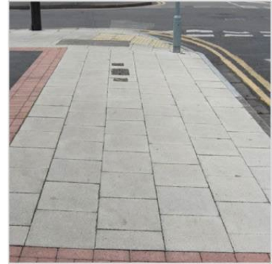
Example of slab footway with decorative edge in good repair.
