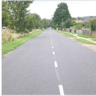
Example of Asphalt Carriageway in good repair.
