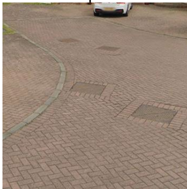
Example of monoblock footway and carriageway in good repair.
